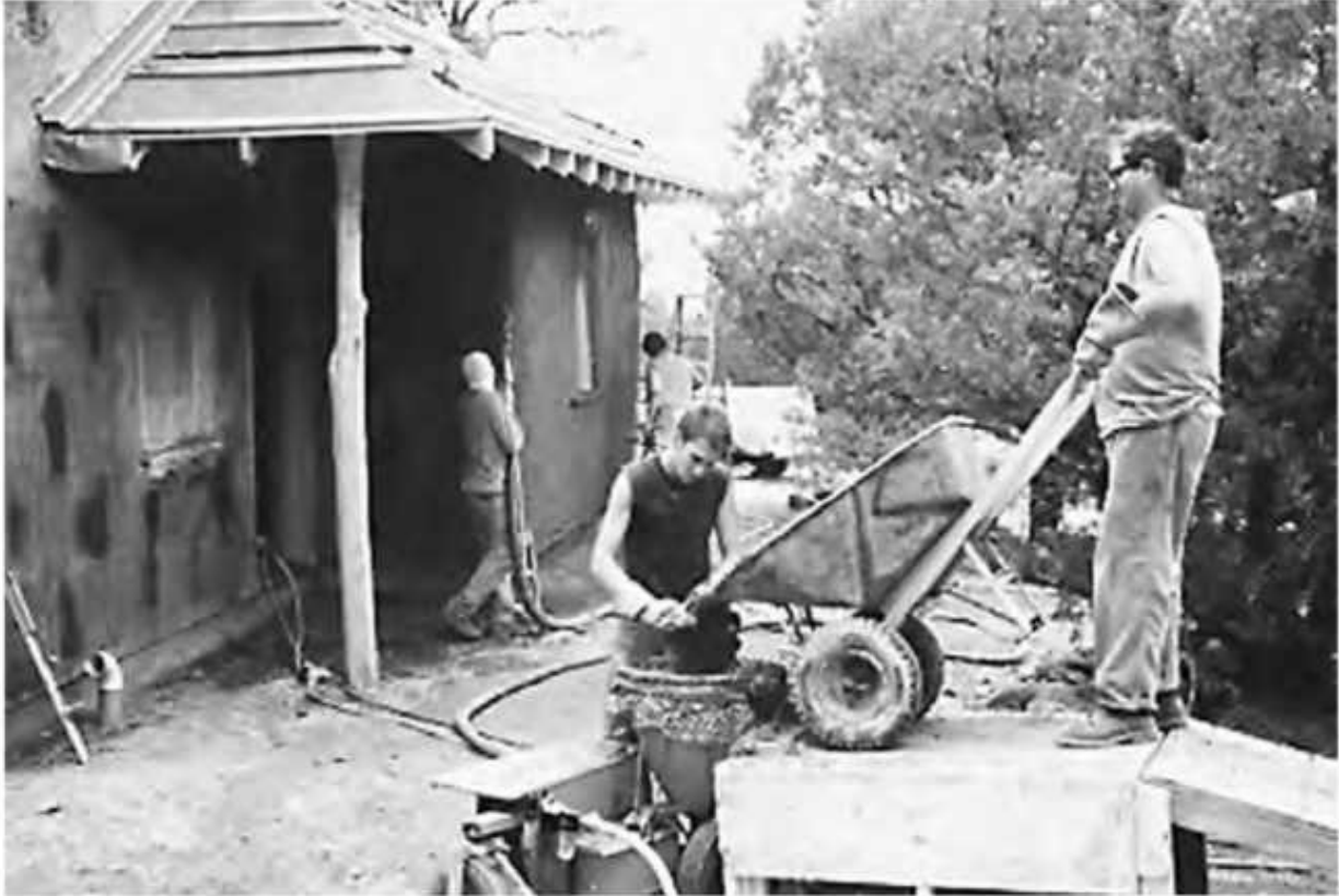
6-24: Workers applying mud plaster using a pneumatic pump sprayer.
