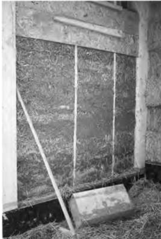
1-17(a) (b): Strawclay is placed in forms, then tamped. When the forms are
