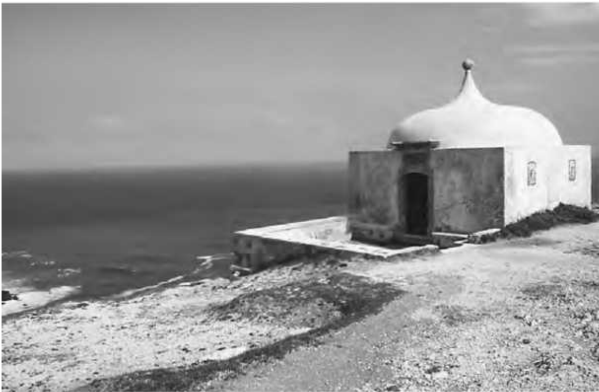
8-1: Lime plaster used on this structure in Sesimbra, Portugal has protected the building for many hundreds of years.
