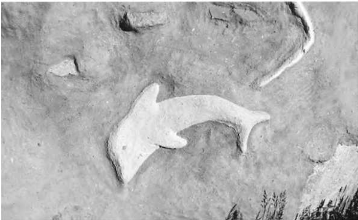
6-16: Earthen plasters are ideally suited to wall sculpting, producing delightful figures like this dolphin or more complex sculptures like the one on the cover of this book.
